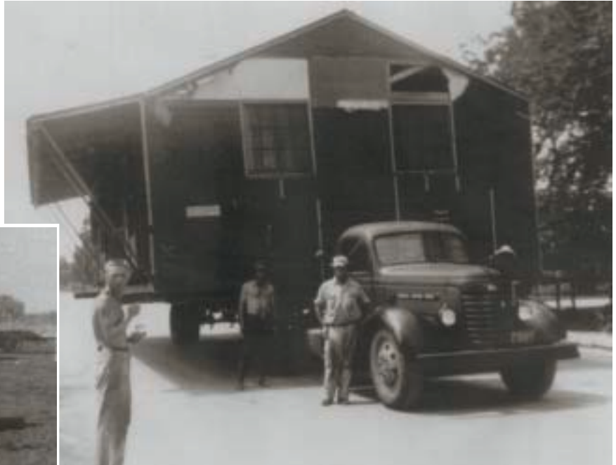
Moving the Labelle, Florida City Hall in 1949. Tom Doyle is in the left foreground with no shirt.
